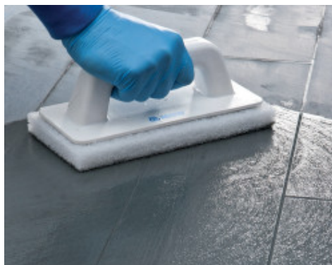
Cleaning the joints with a ScotchBrite® pad (when the product is semi-hardened)
